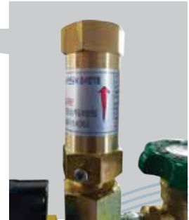
Safety Valve (Discharge Device of Abnormal Pressure)
