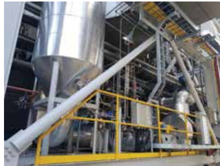
Aqueous Ammonia E-Vaporizer
