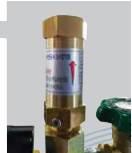
Safety Valve (Discharge Device of Abnormal Pressure)
